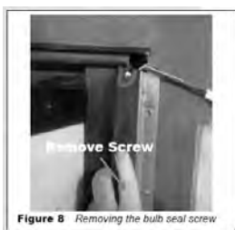
Figure 8 Removing the bulb seal screw
